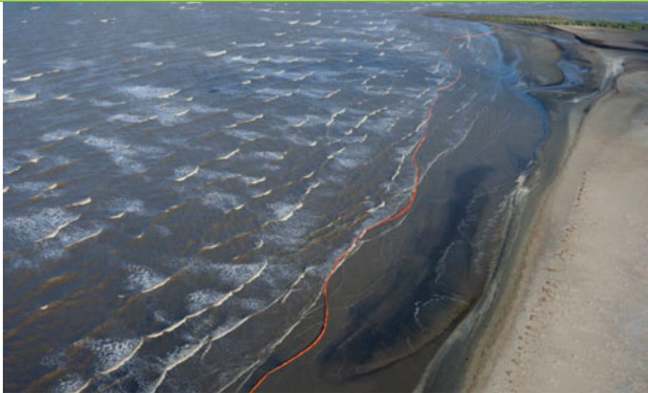
Booms have been deployed in a bid to prevent the flow of oil leaking from the Deepwater rig reaching the Louisiana coastline. Photograph: Liz Condo/AP
